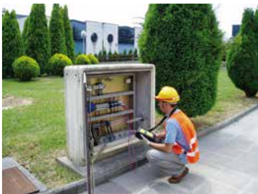
Signal injection in a power-box using the IC1G transmitter (TX)
